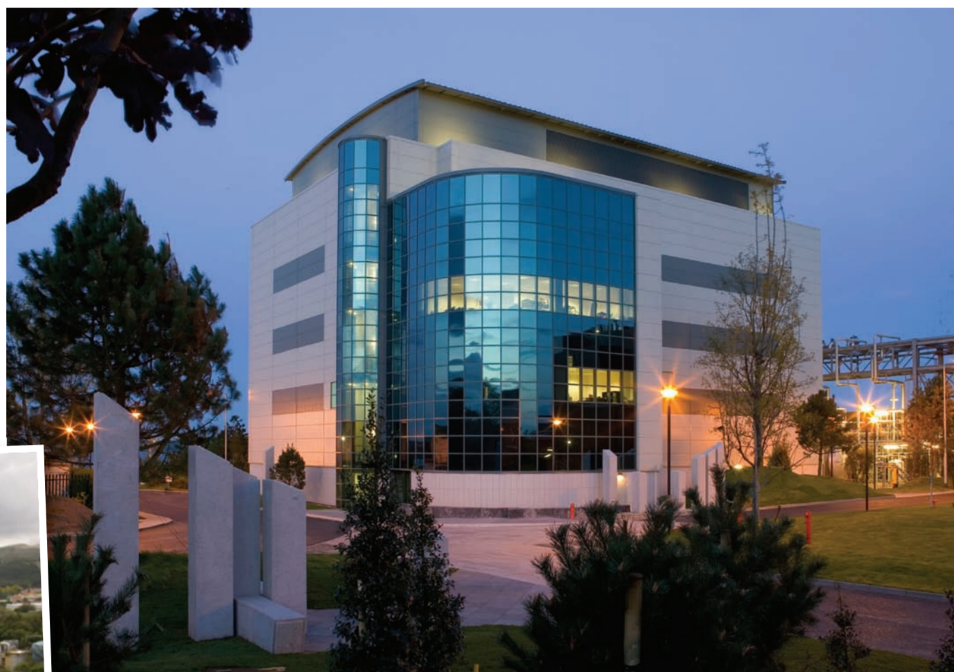
ABOVE: Spray drying building, Cork plant. LEFT: Roger Viney.
